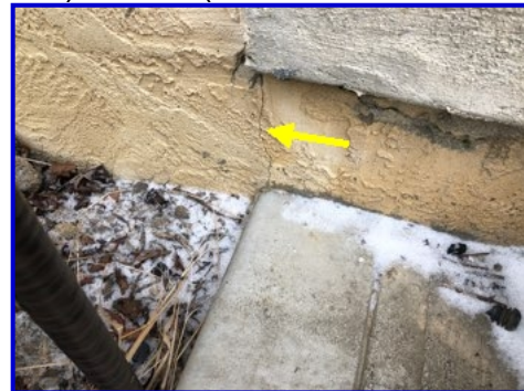
Stucco crack observed (rear of home above patio)
