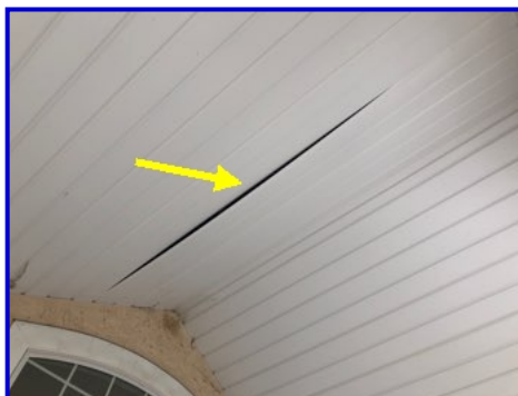
Loose soffit (rear covered porch)
