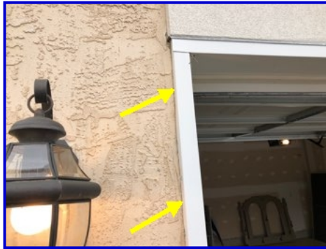
Seal joints of dissimilar materials (around exterior windows)
