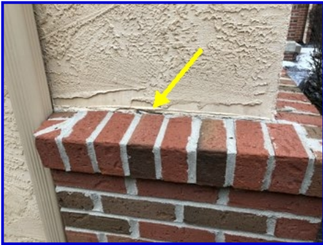
Seal joints of dissimilar materials (Southeast corner)
