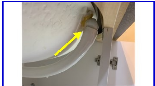
Master sink leaks at overflow connection
