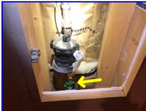
Main water shut off (basement south wall)
