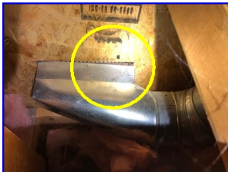
Disconnected vent in (west) crawlspace
