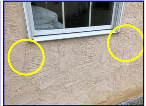
Stucco cracks should be repaired (around exterior windows)
