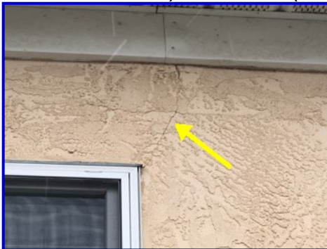
Stucco cracks should be repaired (around exterior windows)
